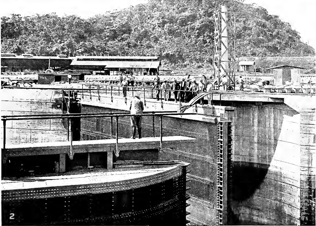
1. Lock gates at Gatun in course of construction. 2. After completion. There are 92 leaves, weighing from 300 to 600 tons each.
